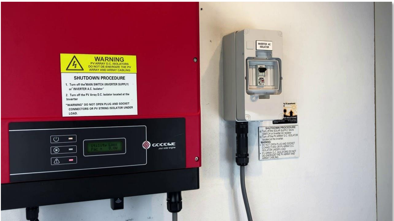
An example of AC Power Supply Switch next to inverter:
