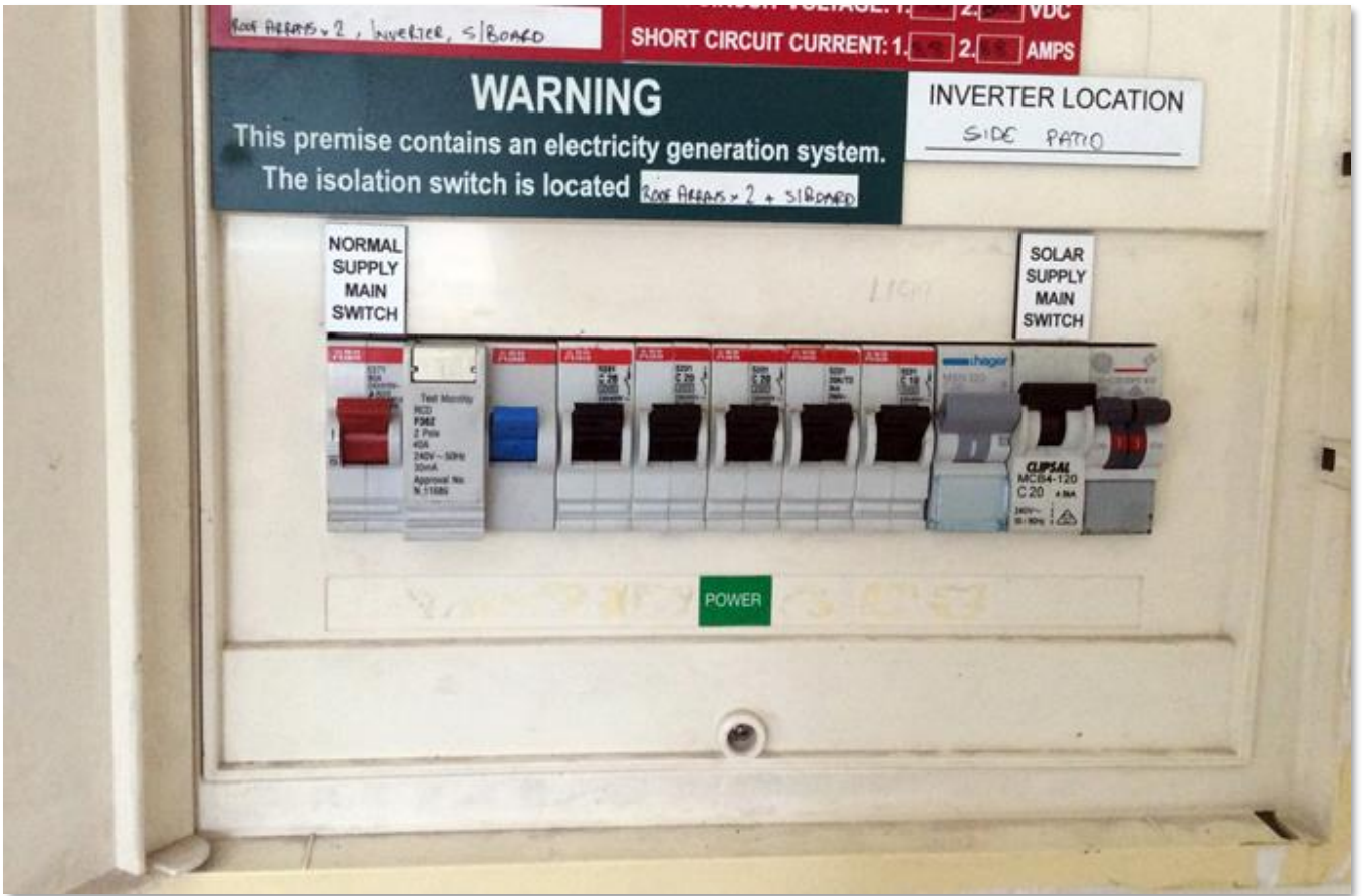
An example of Solar Supply Main Switch on a domestic switchboard:
