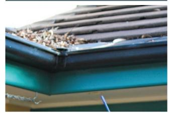
**Explanation** Either direct flame contact or embers can set this litter alight. While the leaf litter is loose, it is aerated and easily flammable. Burning leaves can get under the tiles and into the roof space and spread fire to other parts of the building and property.
