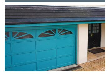
**Explanation Door mat:** Embers can be trapped by the mat causing it to catch fire. Flame and embers from the burning mat can penetrate under the door, introducing fire to the inside of the house.
