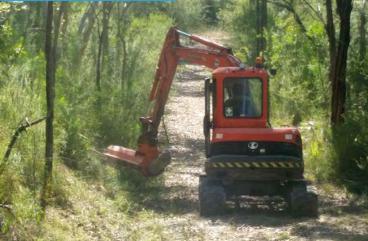
Photo 52 - Removal of excess vegetation using a mulching head.
