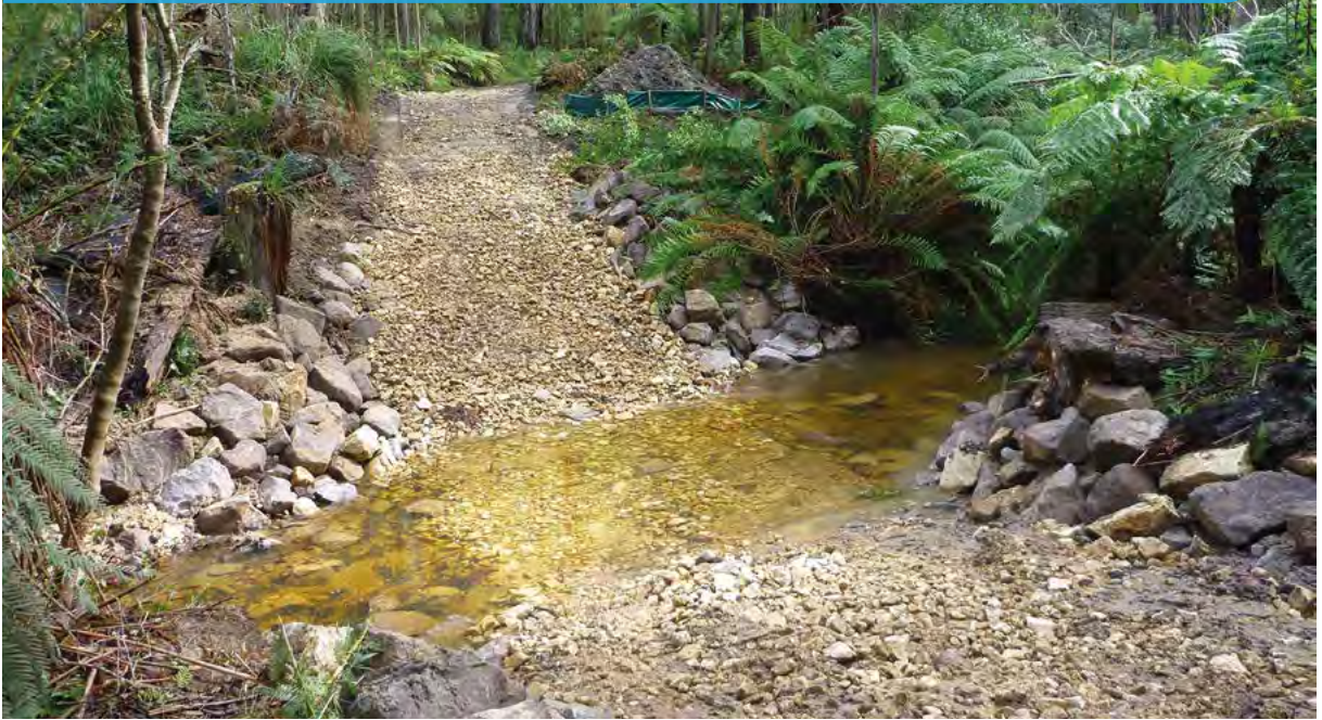
Photo 20 - A bed level crossing/rockfill ford at natural gully floor level. Smaller rock is placed over much larger armour stone that will stay in place in high flows. This bed level crossing has been designed to allow fish passage and will not block or dam the flowline.
