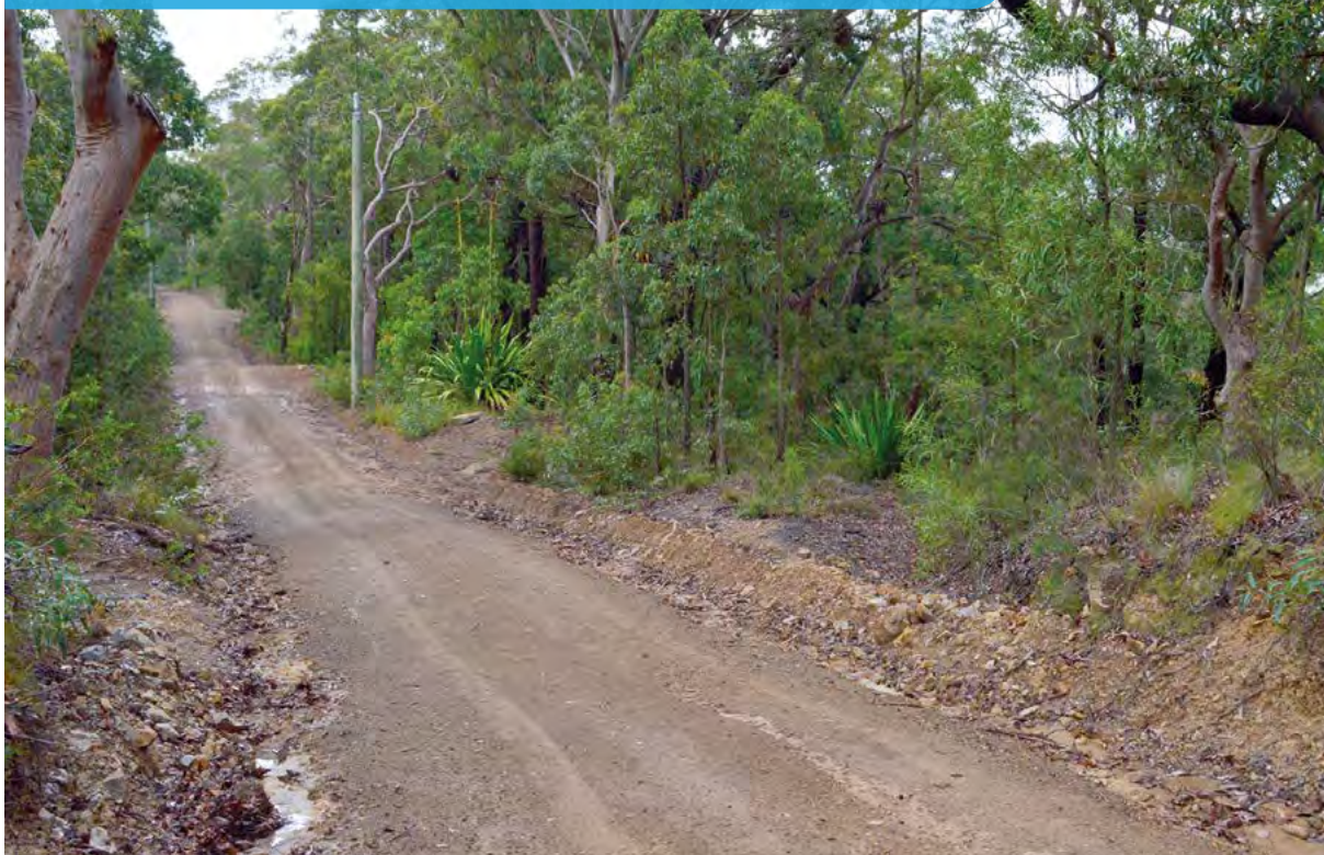
Photo 62 - The reinstatement works have not reformed this existing mitre drain on the right hand side. As a result, flow rates will be too high and cause erosion further down.
