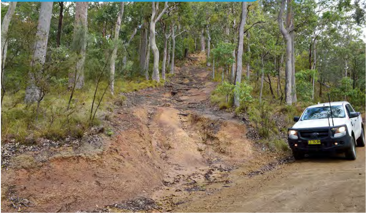
Photo 56 - Unplanned and illegally formed trails quickly erode and cause damage to the environment. The water erodes the formed trail and the sediment blocks drainage structures. These trees will also collapse, causing further soil disturbance.
