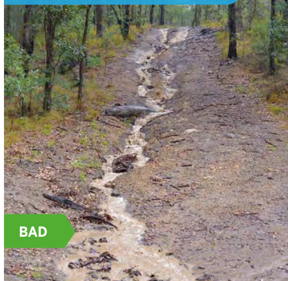
Photo 51 - A poorly constructed and maintained trail will easily erode prevent access and cause environmental damage.
