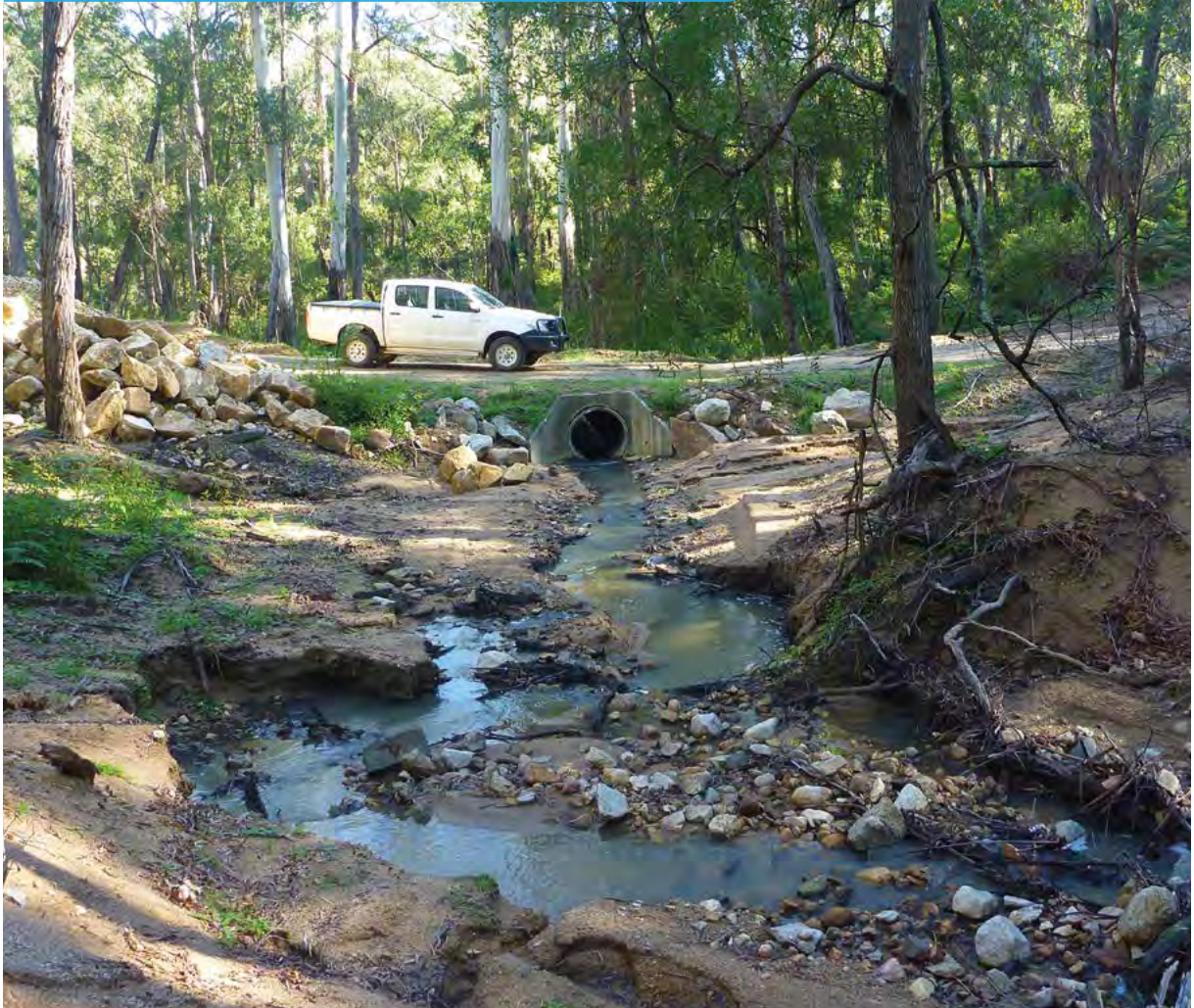
Photo 34 - This culvert is too small and therefore prone to blocking, which will damage the trail. A rock armoured bed level crossings is a better alternative.
