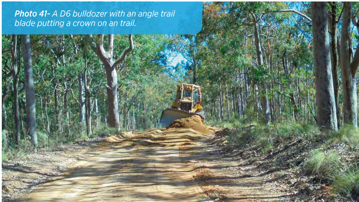
Photo 42 - D6 bulldozer capping and crowning a trail.
