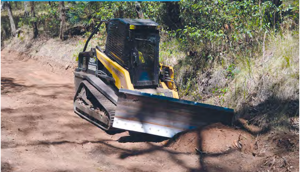
Photo 54 - Maintenance of table drains a 100HP skid steer with tilt blade cleaning out table drains.
