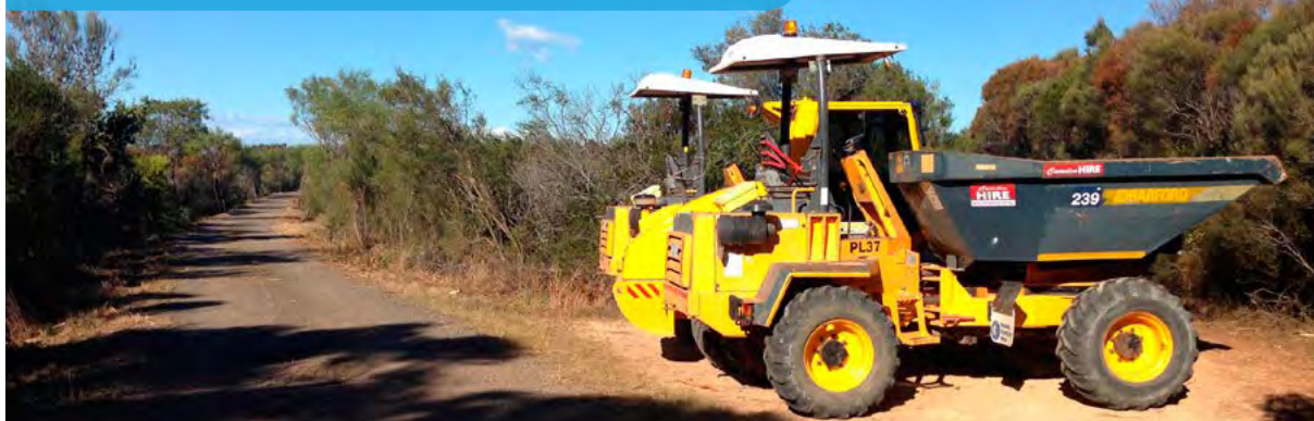
Photo 35 - A durable VENM shale quarried material supplied by a local quarry supplier for a trail surface.
