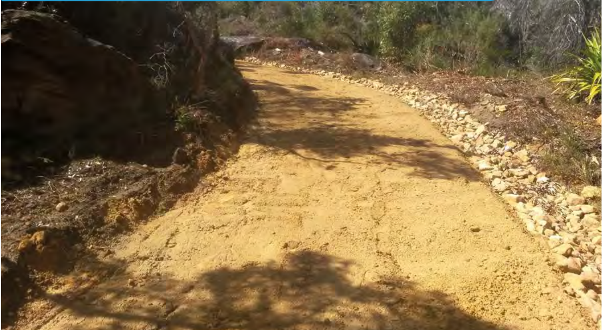
Photo 11 - An outfall on a re-established and previously highly eroded trail. This trail includes a rock lined table drain as these soils are highly erodible.
