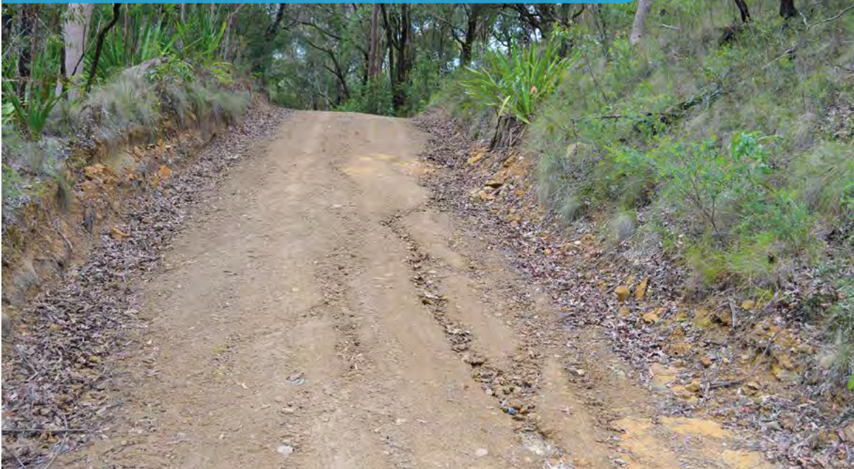
Photo 60 - This trail is too narrow and the table drain on the right hand side has not been formed properly. It blocked easily, causing water to be redirected onto the trail and led to erosion.
