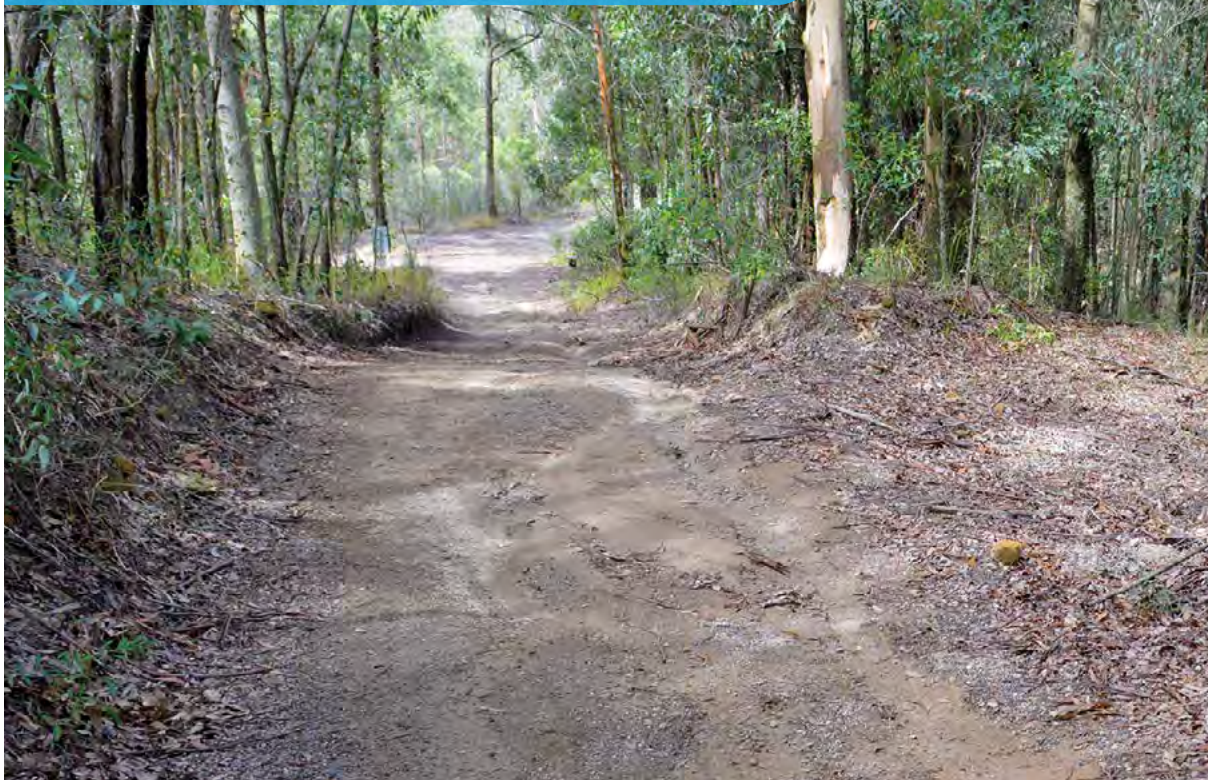
Photo 61 - The new works shown have failed to reinstate the existing mitre drain on the right, hence flows are too large and are eroding the bottom of the trail.
