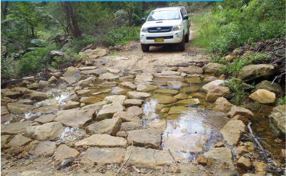
Photo 23 - Rock and stone paving allows access across a wet flow line
