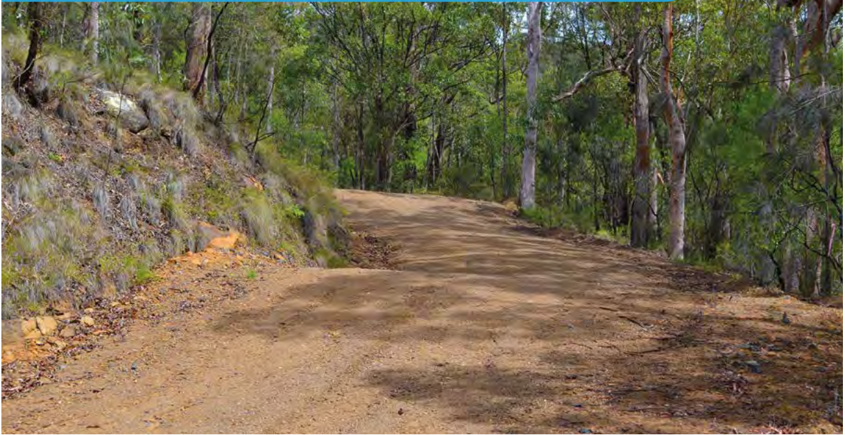
Photo 10 - Outfall drainage. This section of trail is subject to a large catchment on the left. To help drainage there is no windrow on the right downslope of the trail. This allows clear unrestricted outfall of drainage water. Note there is no batter fill on the right downslope side.
