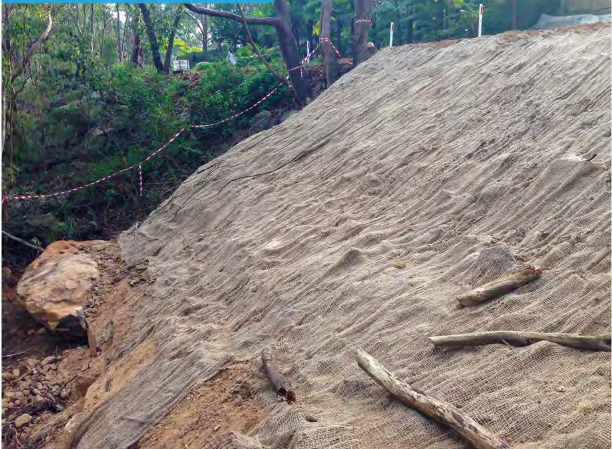
Photo 36 - A batter slope protected with jute mesh on an infall trail.
