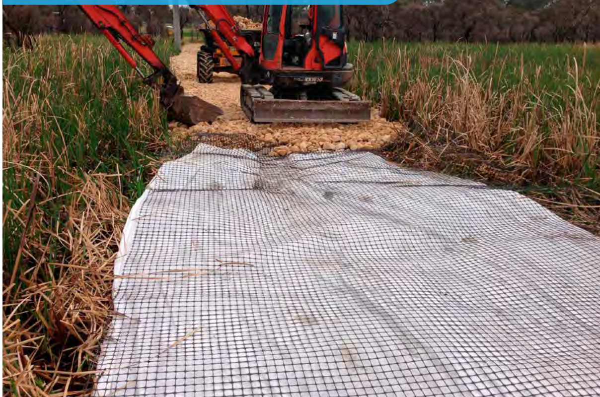
Photo 26 - Using Geotextile cloth, plastic geomesh and rock to construct access across a very wet area.
