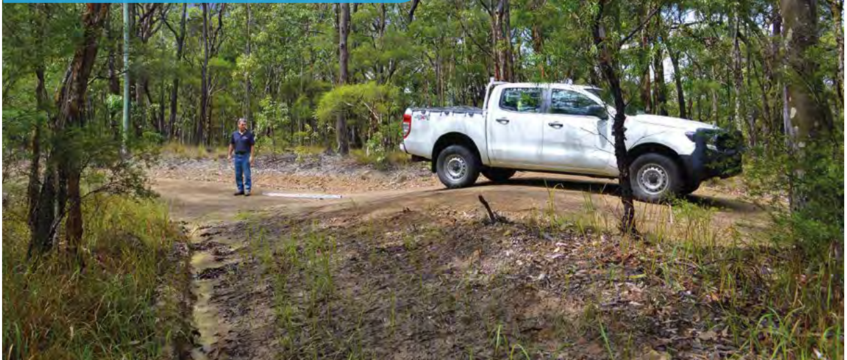
Photo 14 - A cross bank directing runoff across the trail surface to a mitre drain.
