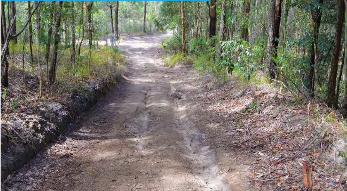
Photo 59 - A poorly constructed trail with no crown or table drains, repaired only 18 months ago. The newly formed gullies will soon make this trail impassable.
