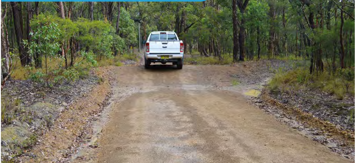
Photo 15 - A cross bank directing runoff across the trail surface and into a mitre drain.
