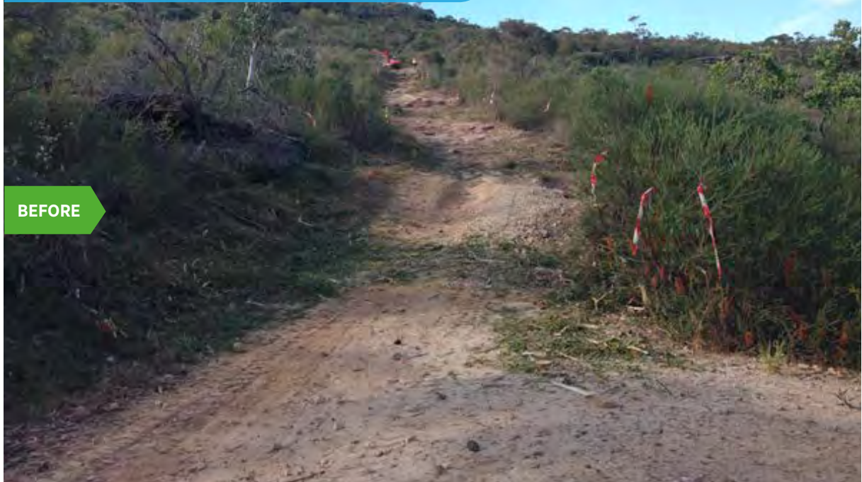
Photo 39 - After clearing the trail of vegetation, before constructing the trail surface.
