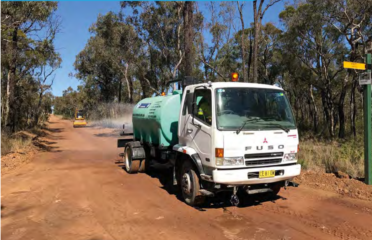
Photo 44- The addition of water and a roller greatly improve compaction, particularly if conditions are dry.
