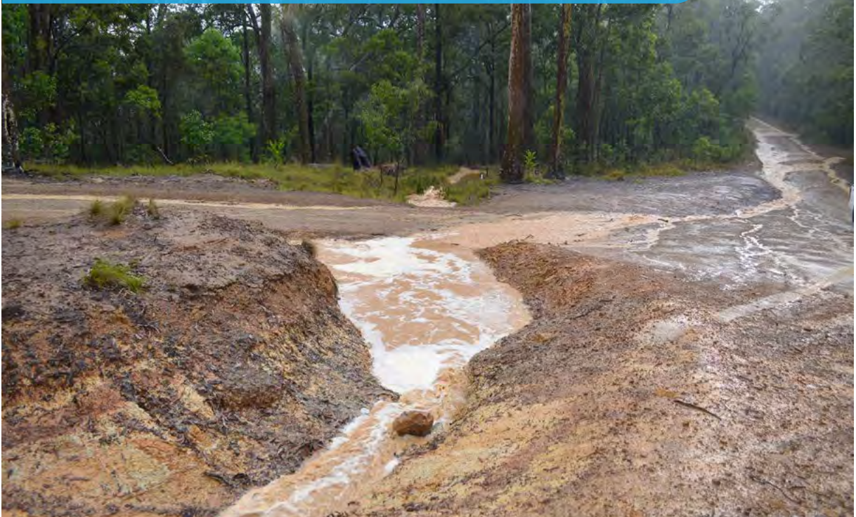
Photo 32 - This blocked culvert is redirecting and concentrating drainage down the formed trail and causing erosion. Drainage using cross banks and open rock paved spoon drains is a better option.
