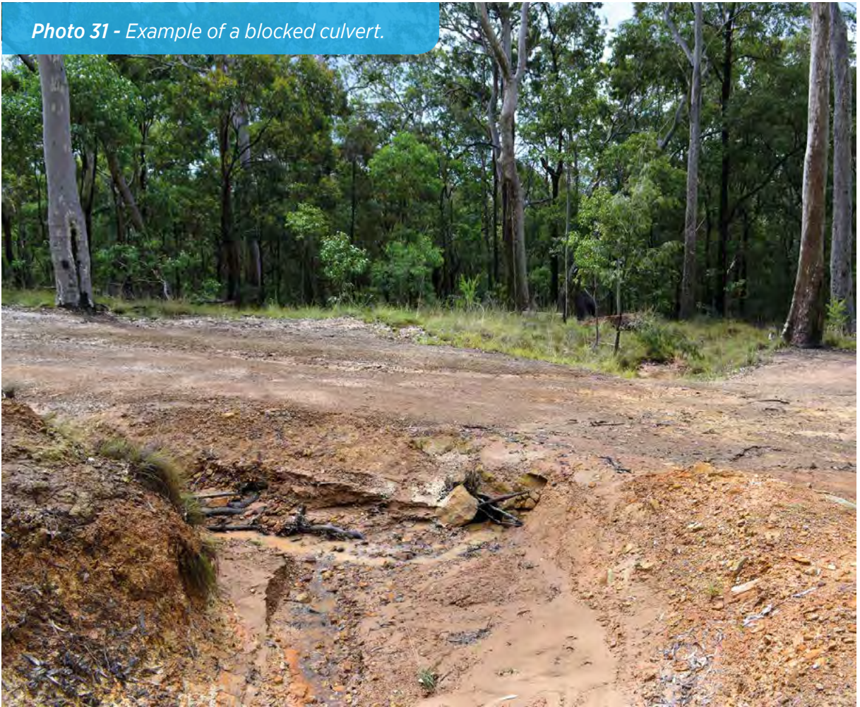
Photo 32 - This blocked culvert is redirecting and concentrating drainage down the formed trail and causing erosion. Drainage using cross banks and open rock paved spoon drains is a better option.
