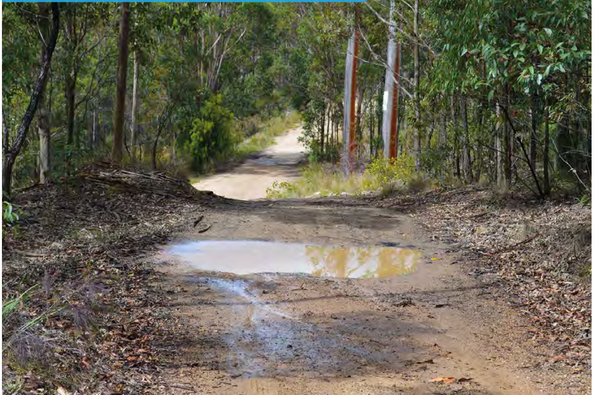
Photo 65 - This trail should be crowned to shed water. There should be no pooling of water on the trail.
