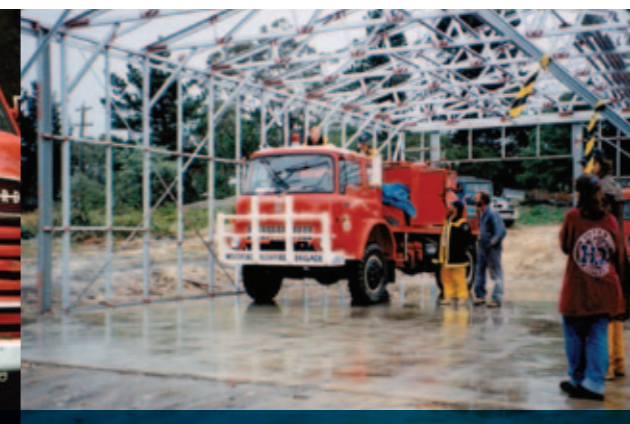
1995: Building the extensions
