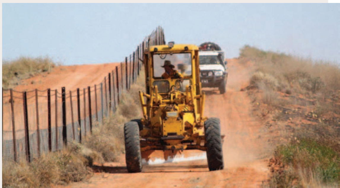
ABOVE: A grader working along the dog fence, building containment lines on the NSW/SA border. Photo by Mark Lacy.
